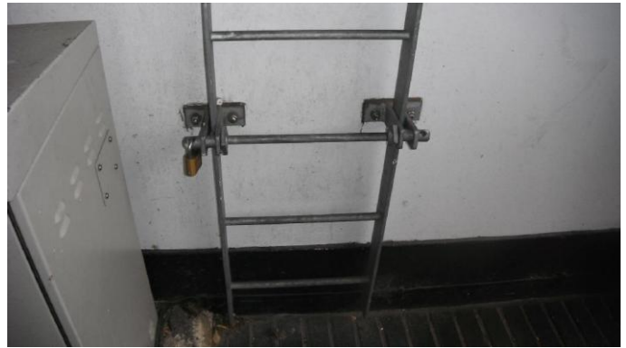
Secured access ladder
